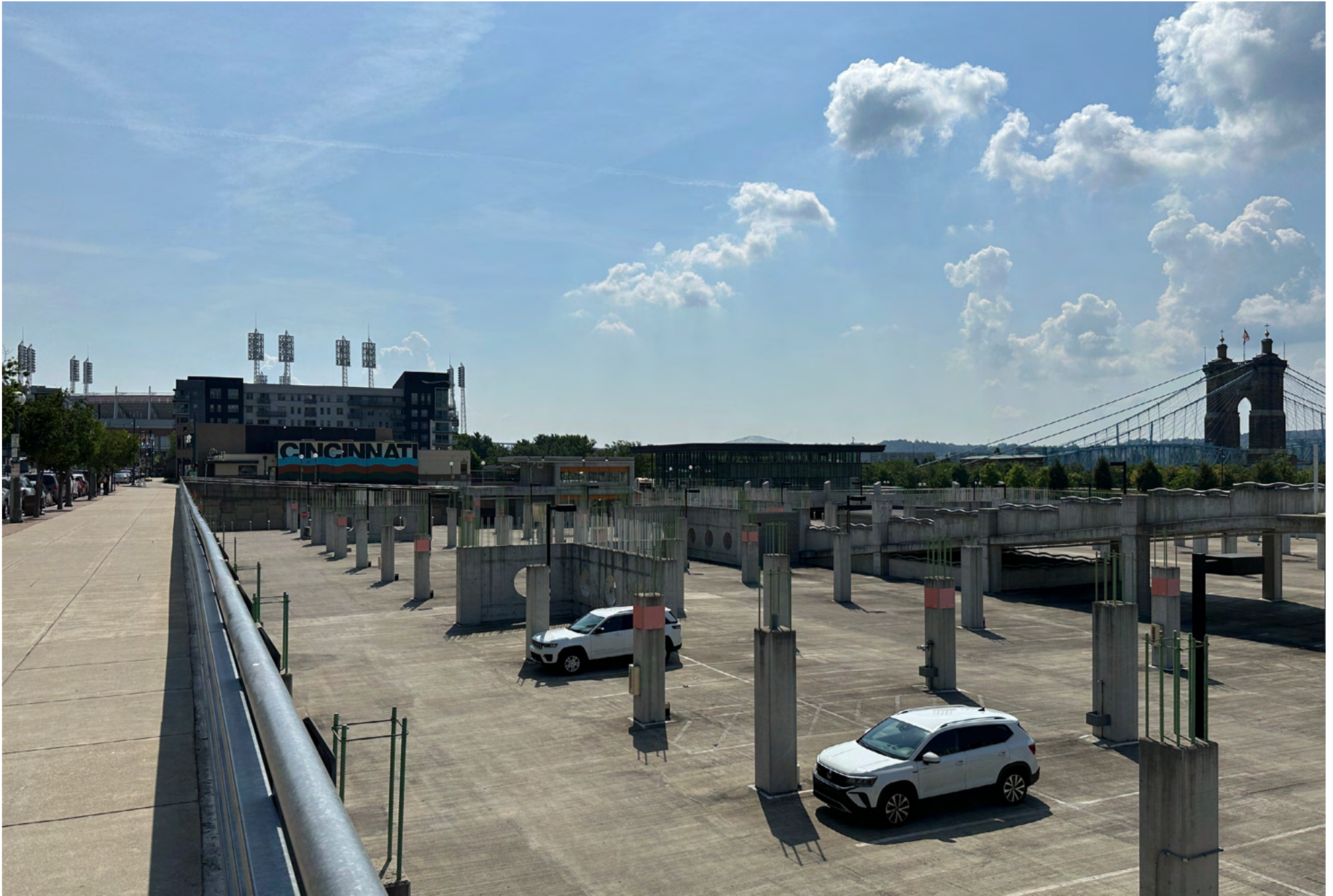
ABOVE Lot 24 looking toward Roebling Bridge
