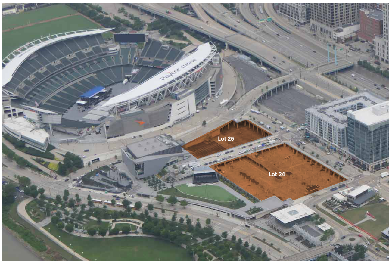
Aerial Image, Banks Public Partnership
